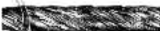
Infrequent inspection. Neglect of periodical inspection left this rope in service too long, resulting in considerable abrasion.
